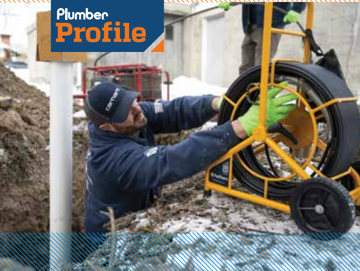
◀ Frank Roberts sets up the Hathorn camera reel for job site usage.
